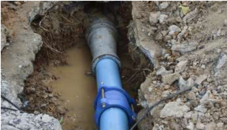
Dedicated coupling on PVC replacement pipe
