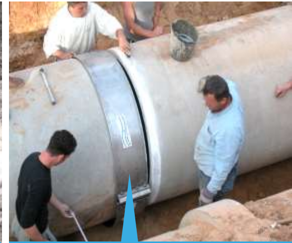
Hydraulic wide-range openable Coupling in a joining function
