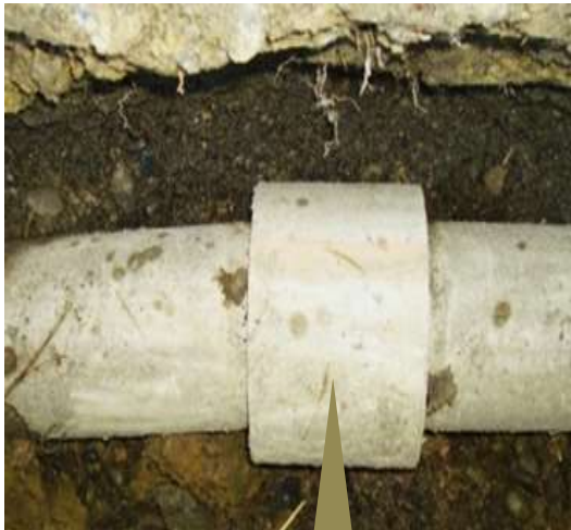
Original asbestos coupling
