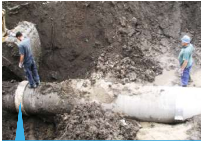
Hydraulic wide-range openable Coupling in a repair function
