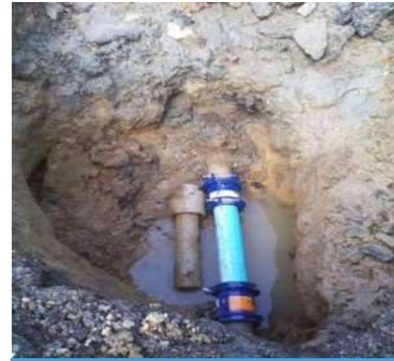
Wide range couplings on PVC replacement pipe
