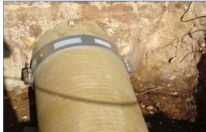
Wide-range openable Coupling
