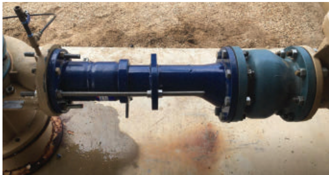
The Queen Creek utility was able to replace rusted sections of its pipeline system without using tailored pipes for each repair.
